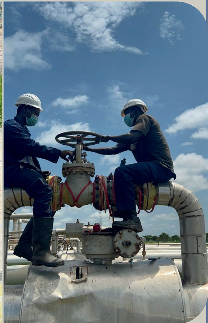
Figure 12: above ground work
