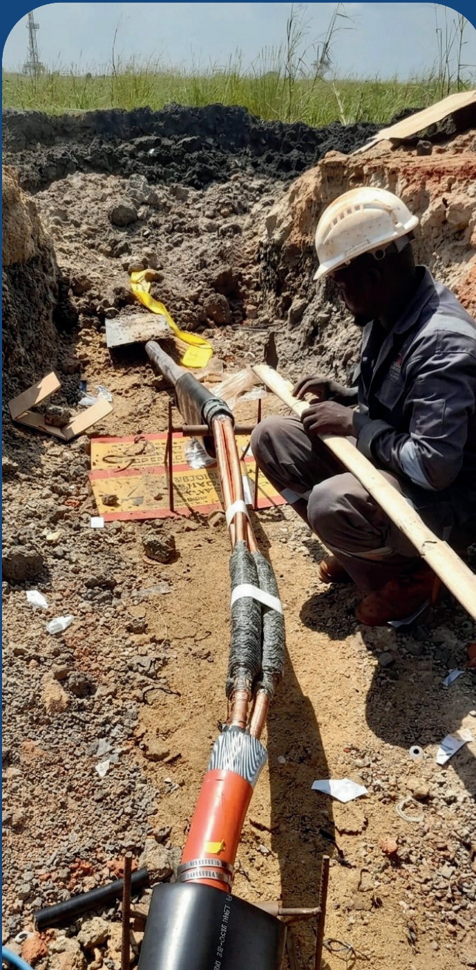
Figure 5: cable termination.
