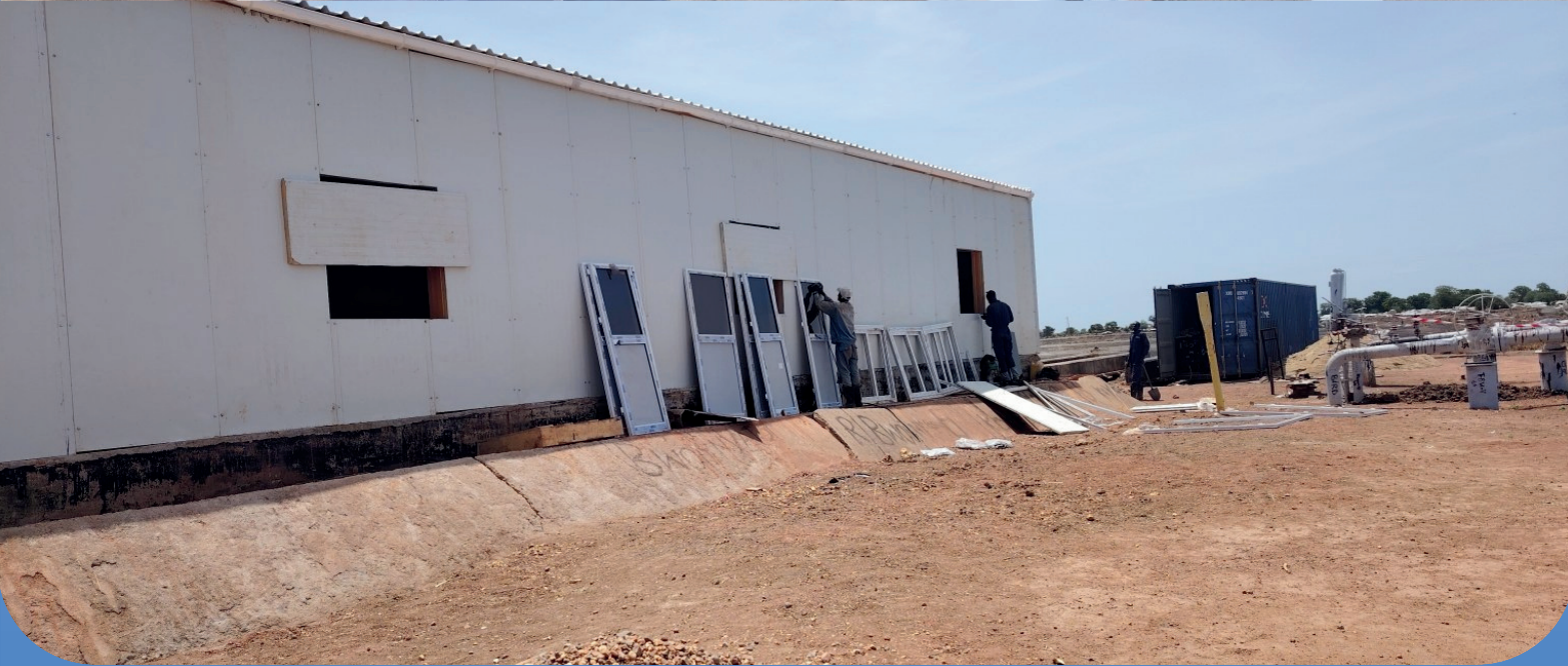
Figure 19: BVS-1 fabrication and the building
