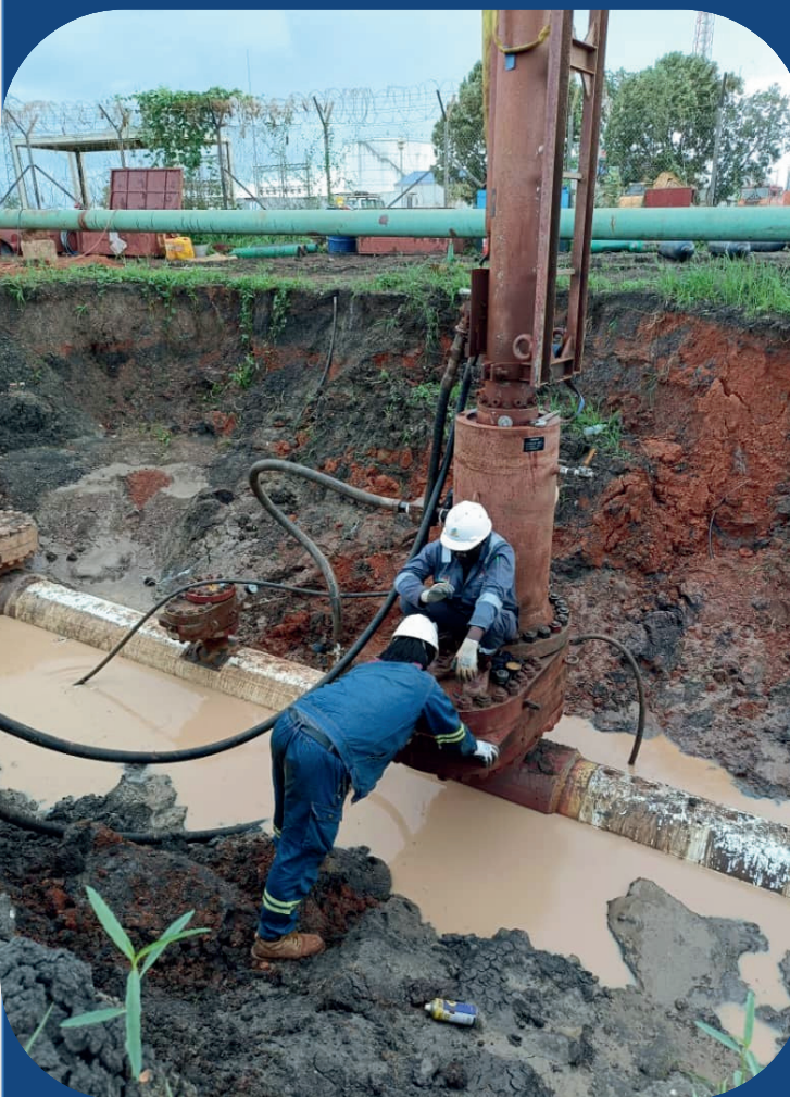
Figure 9:connecting sandwich valve
