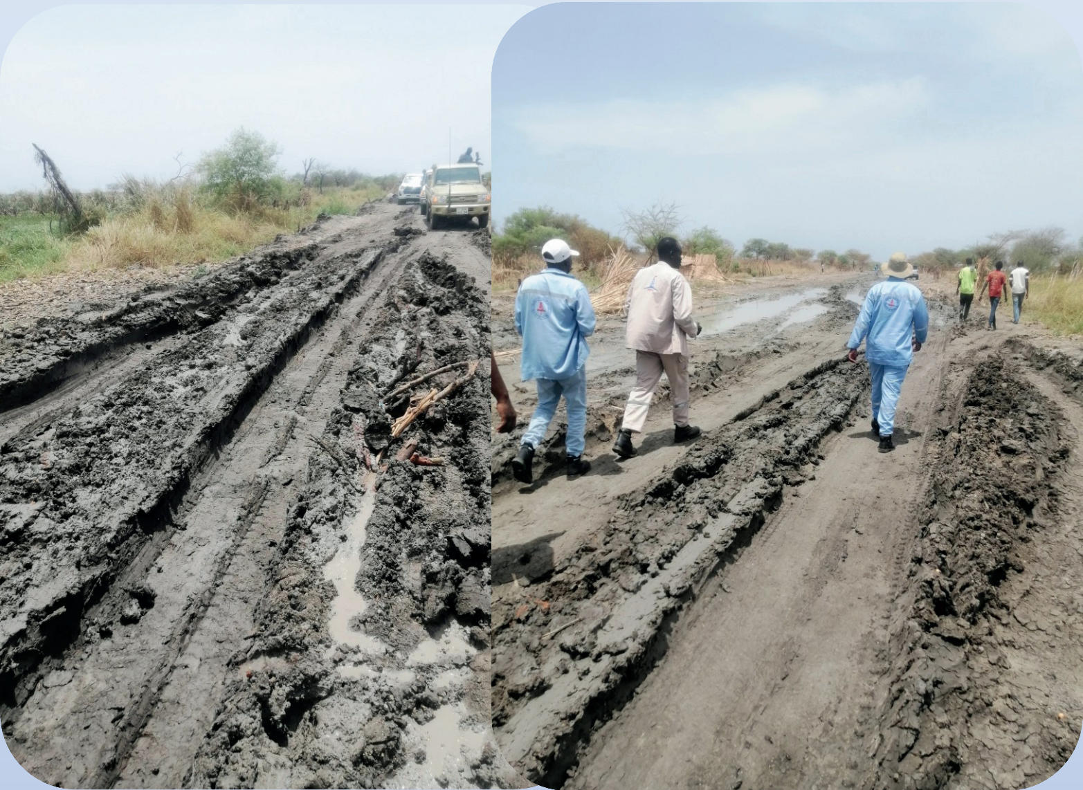
Figure 18: Road construction is going on
