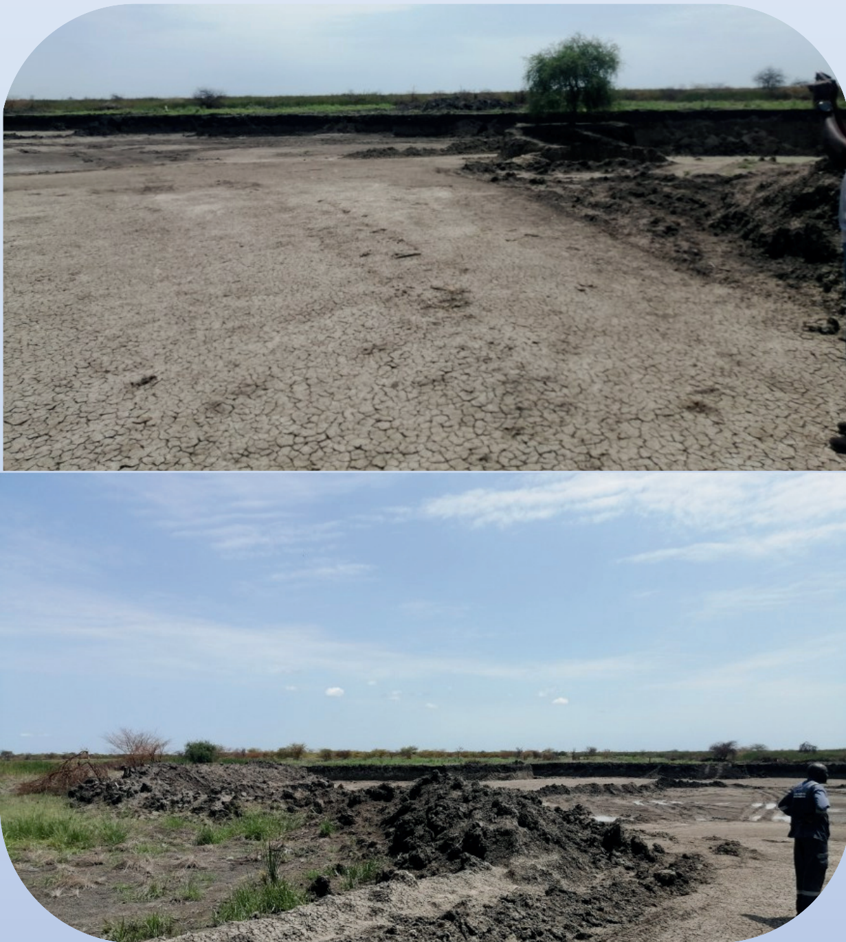
Figure 16: Lake No road construction
