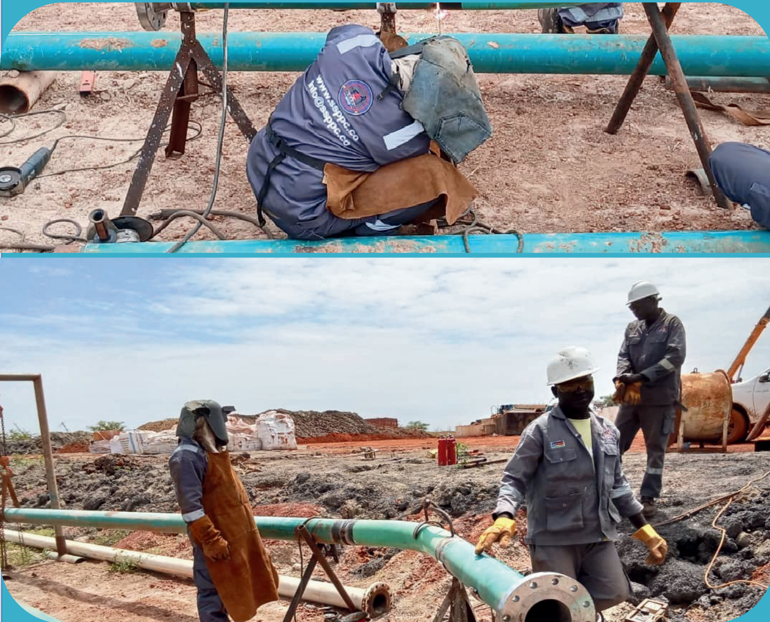
Figure 4: joint welding for new infill well flowline by certified 6G welders.
